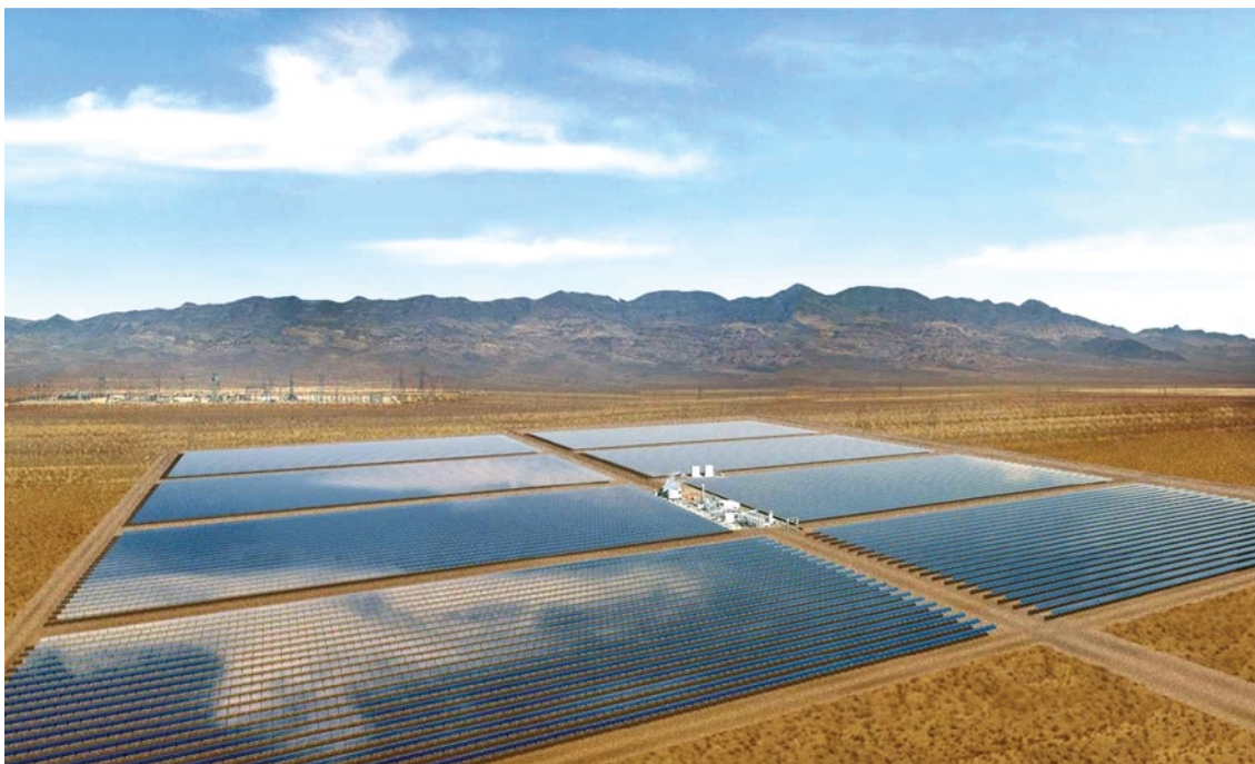
Figure 4: The solar thermal energy plant in Eldorado Valley, Nevada
