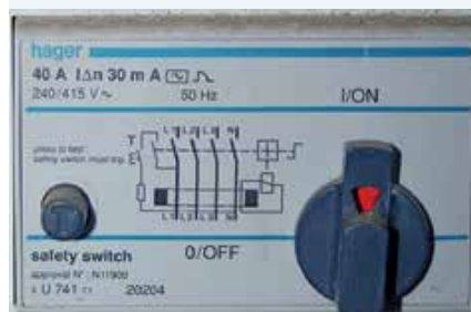
A safety switch, also called a residual current device
