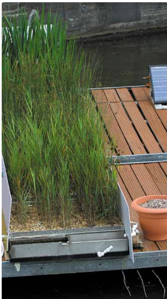
A reedbed is one way of treating greywater.
