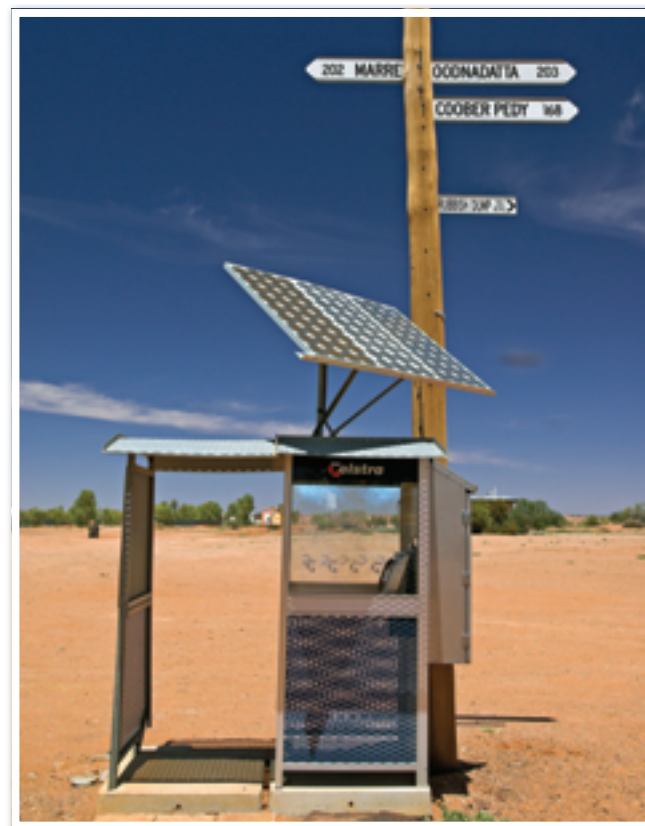
Fig 6.4.7 Solar cells are extremely useful in remote areas where it is too difficult or too expensive to install power lines.
