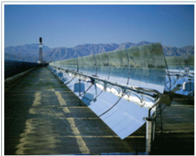
Fig 6.4.9 Computerised mirrors track the Sun and focus its heat and light onto the same point on the Winston tube.
