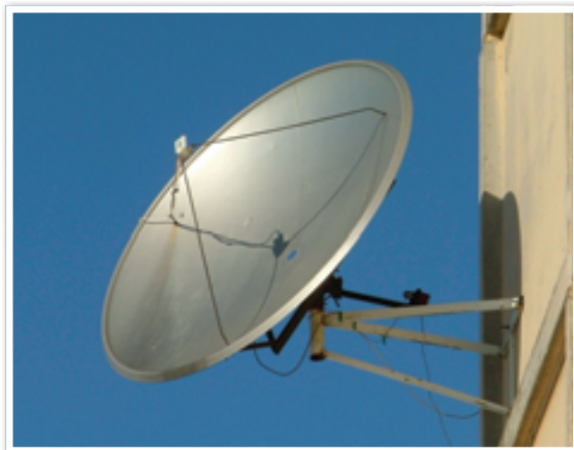
Fig 9.4.5 Most communications satellites (for telephone, TV etc.) orbit so that they are always located over the same point on Earth. This allows satellite dishes to be fixed in the direction of the satellite. If the satellite was in some other orbit, the dish would need to 'track' the satellite to keep in contact with it.
