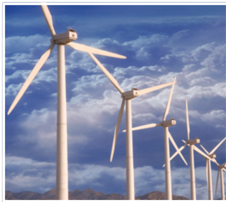
Fig 6.4.12 Wind farms are already becoming a common sight along Australia's coastline.
