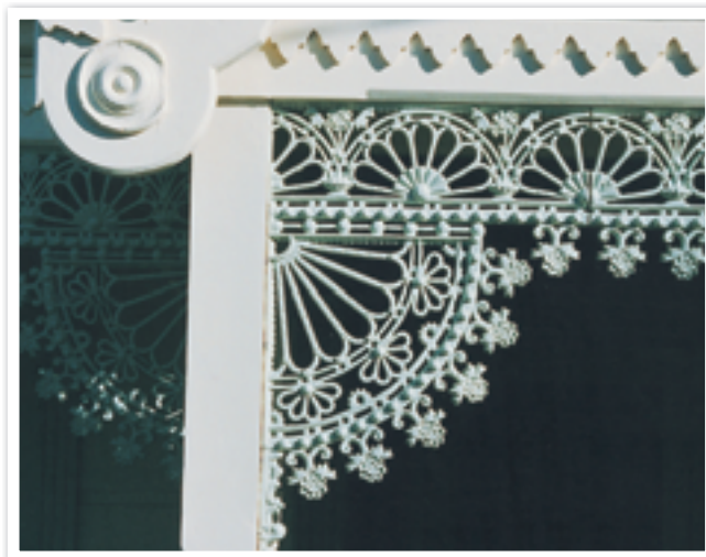
Fig 2.1.4 Cast iron lace is very hard and very brittle.
