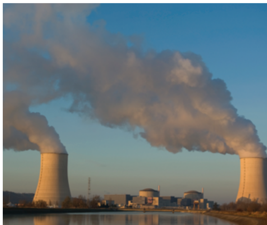
Fig 8.3.1 A nuclear power station and its cooling towers
