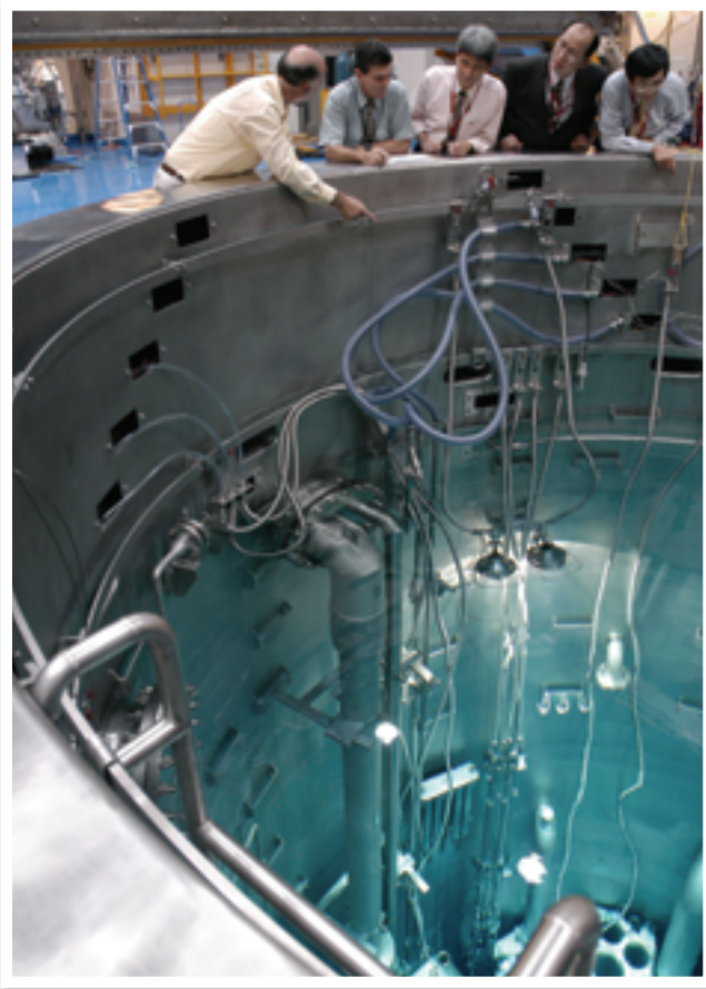
Fig 8.3.7 Australia's nuclear research reactor at (ANSTO) the Australian Nuclear Science and Technology Organisation
